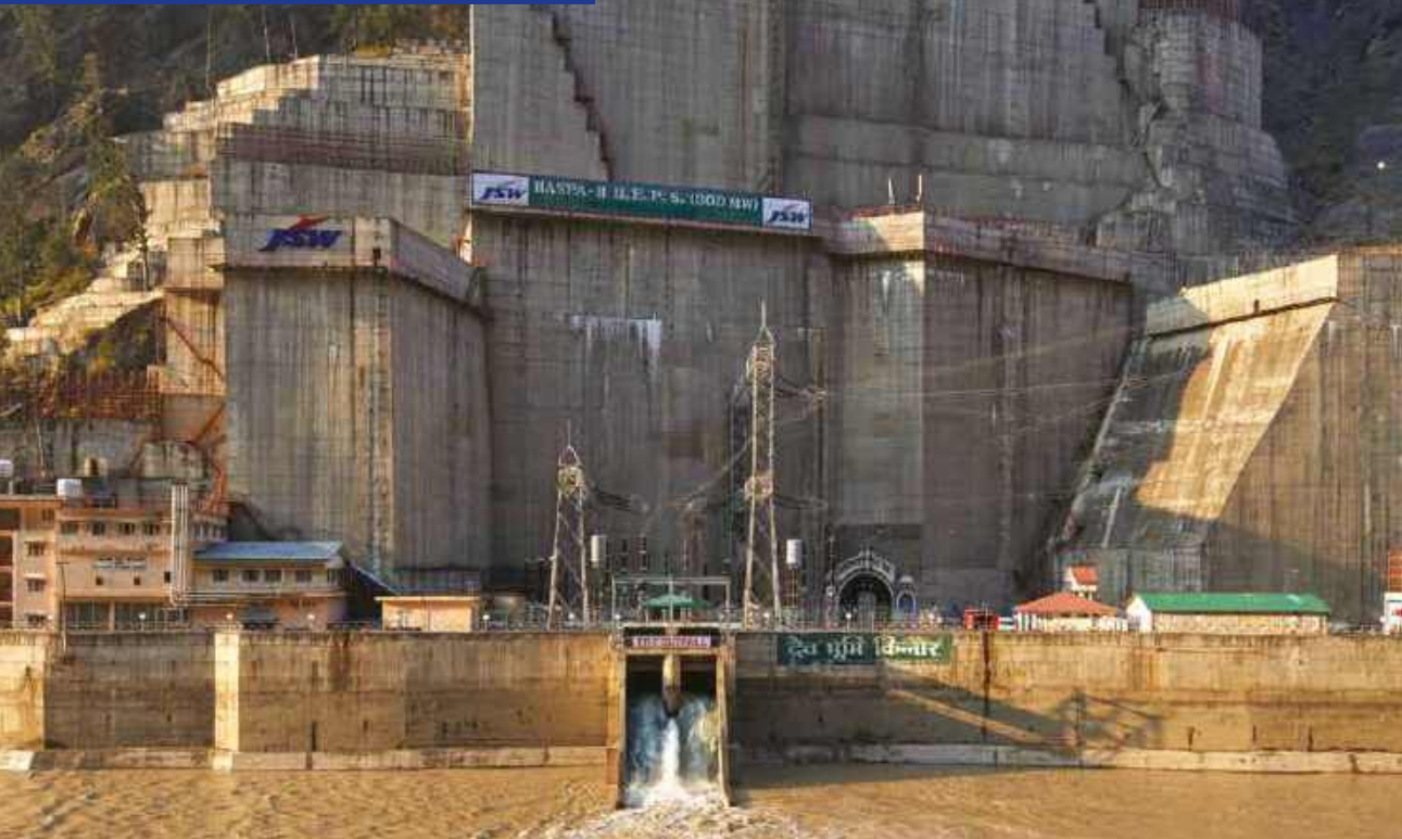
— Baspa-II Hydro Plant, Sholtu
