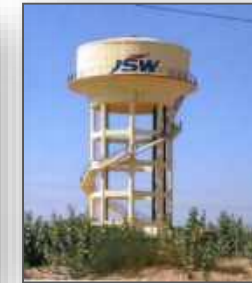
Piped Drinking Water supply to 440+ household near Barmer
