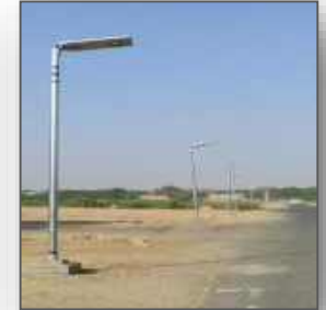
Installation of 371 solar street lights in 4 Gram Panchayats
