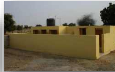
Swachh Bharat Mission: Construction of ~150 individual, community & school sanitation facilities
